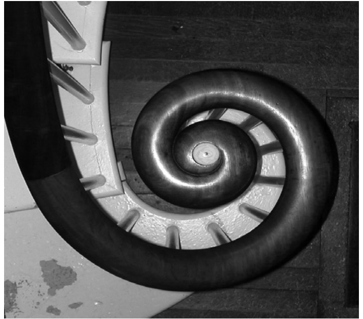
Detail of the volute shaped ease-off at the end of the flying staircase at Woodlawn.
