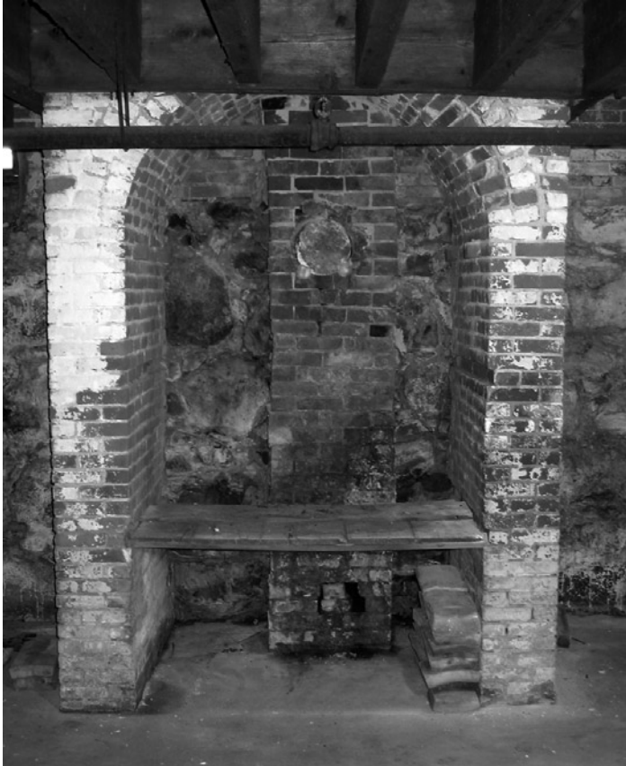
Brick arch supporting parlor fireplace at Woodlawn.
